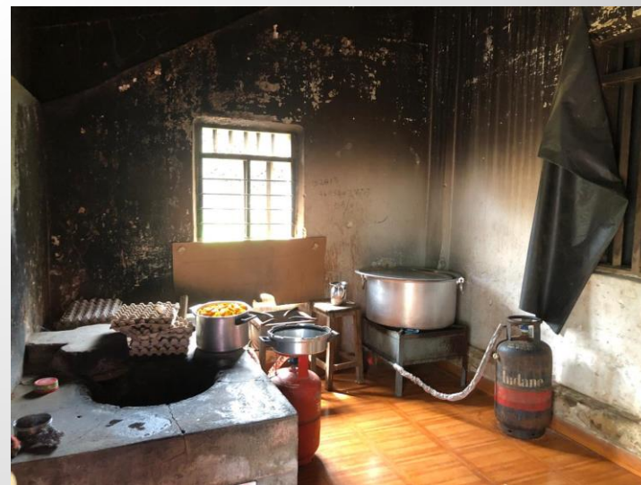
Kitchen Renovation : Rs. 1.5 lakhs
